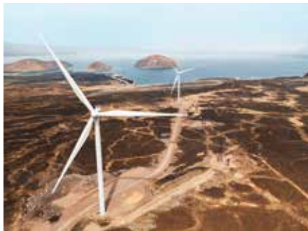
Above and opposite: The Red Sea Power wind farm near the Bay of Ghoubet, 120 km north of the capital
